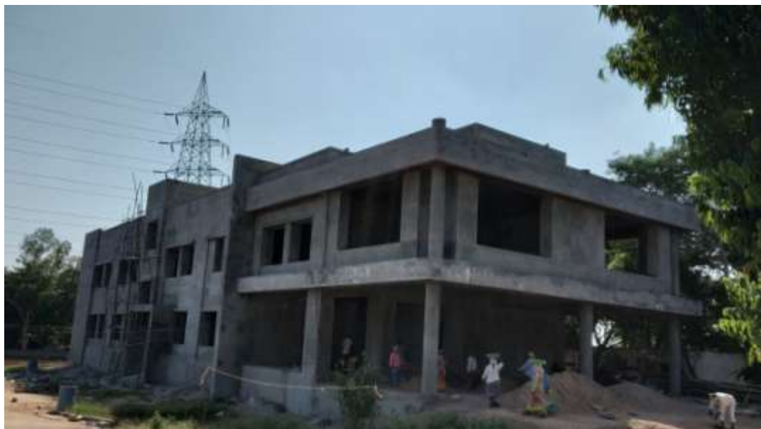
Present status of construction of STL in Rajendranagar
